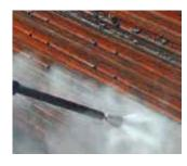
Heavy-duty high pressure water blasters offer powerful and cost efficient cleaning for professional users. Removing paint, rust, markings and graffiti on steel and concrete surfaces.
